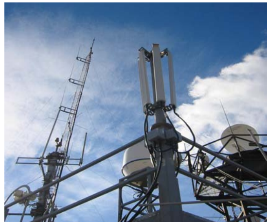
17dBi sector antenna in diversity array
